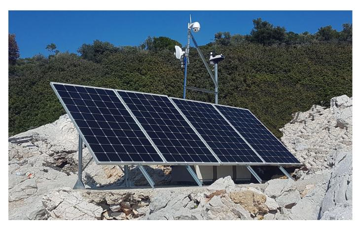
In terms of communications, these are wireless of three types. WiFi communication at a frequency of 5 GHz is currently the main form of interface with the remote control station and is carried out via a point-to-point link between Peristera and Steni Vala.
